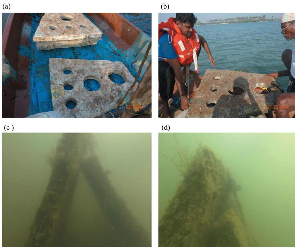
Fig. 18. Adaikkathevan seashore artificial reefs. (a) Artificial Reef in boat (b) Reef step down from boat (c) Placed in Ocean (d) Growth of algae in reef
